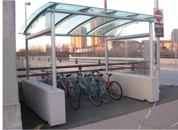
Figure 7.3 – Sheltered Bicycle Parking
