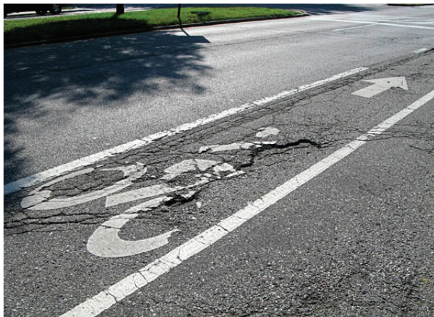
Figure 8.2 – Poorly Maintained Bicycle Lane
