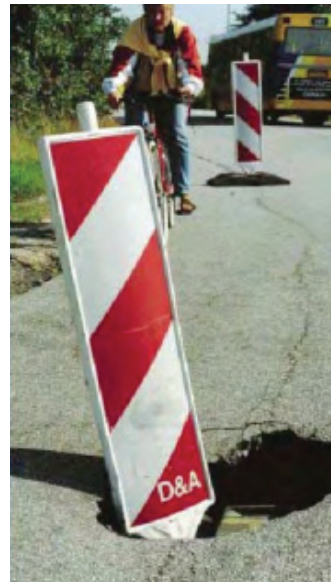
Figure 8.4 – Pothole Identified by Hazard Marker
